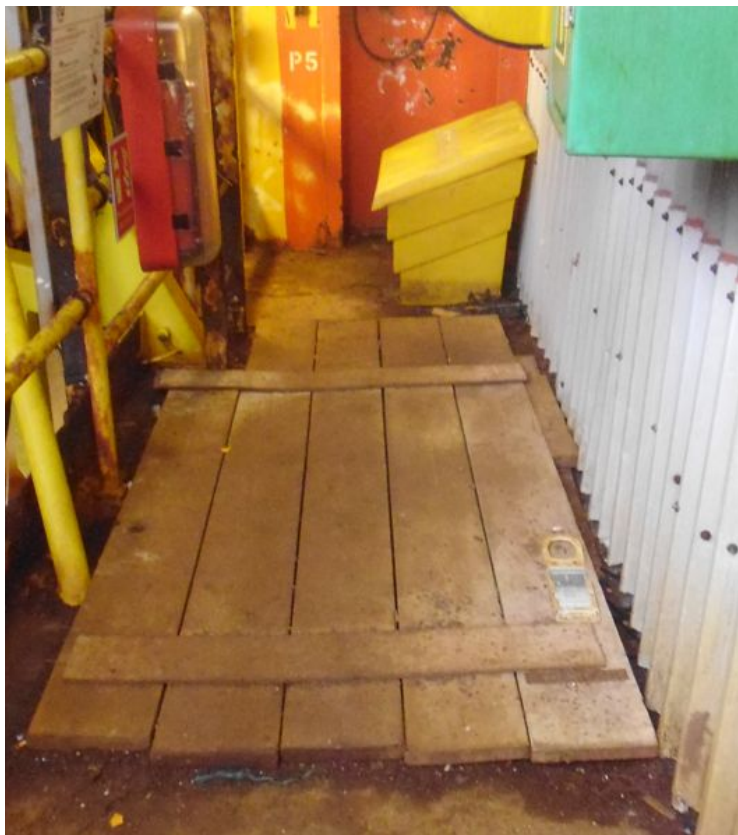
Scaffold boards covering degraded deck plate
