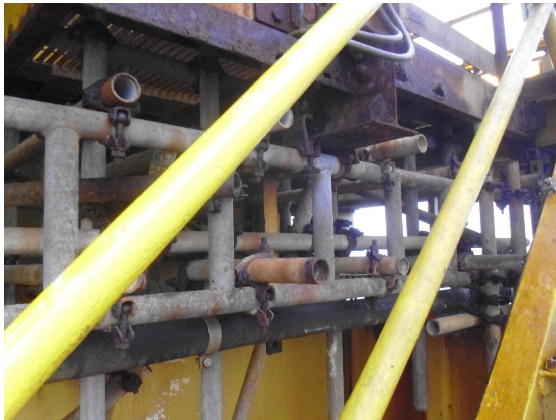
Scaffold supporting degraded structures
