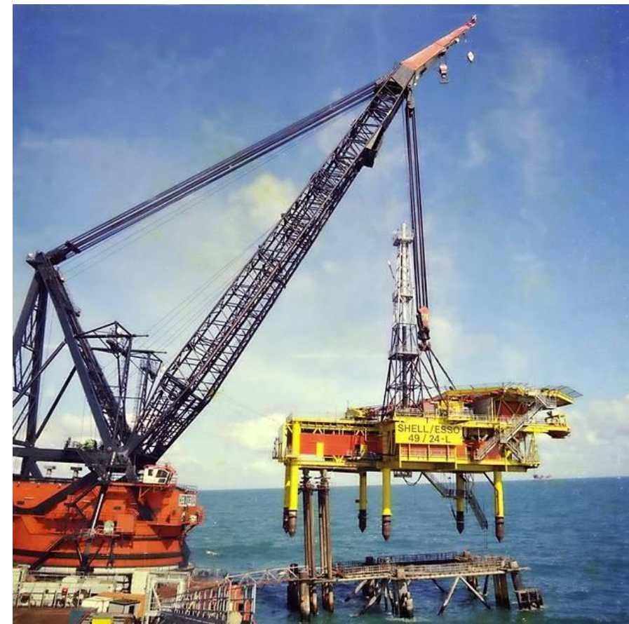
Decommissioning of Shell/Esso Lima platform (Oil Salvage Ltd, 2024)
