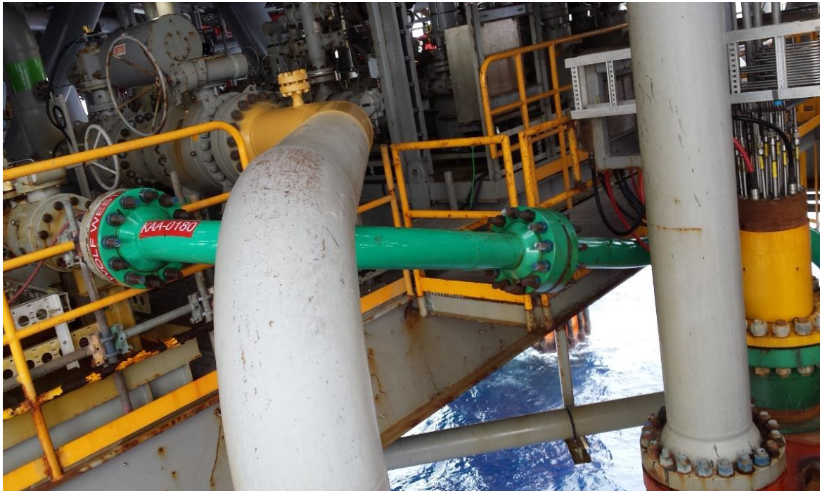
Production piping entering Boarding Valve Skid (prior to installation of IRVS)
