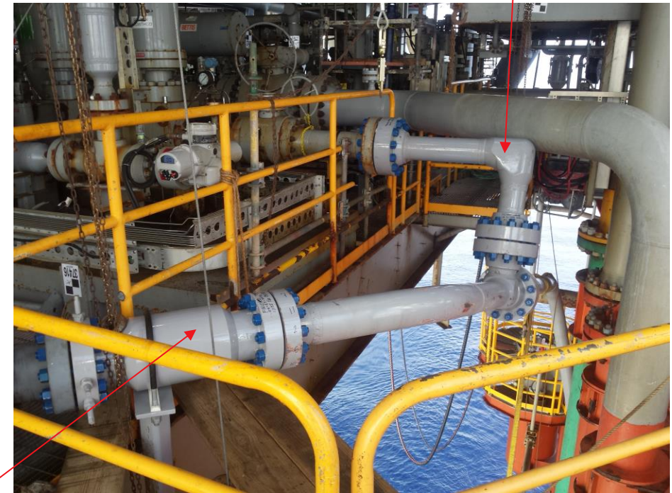
Production piping Modifications (post installation of IRVS)
