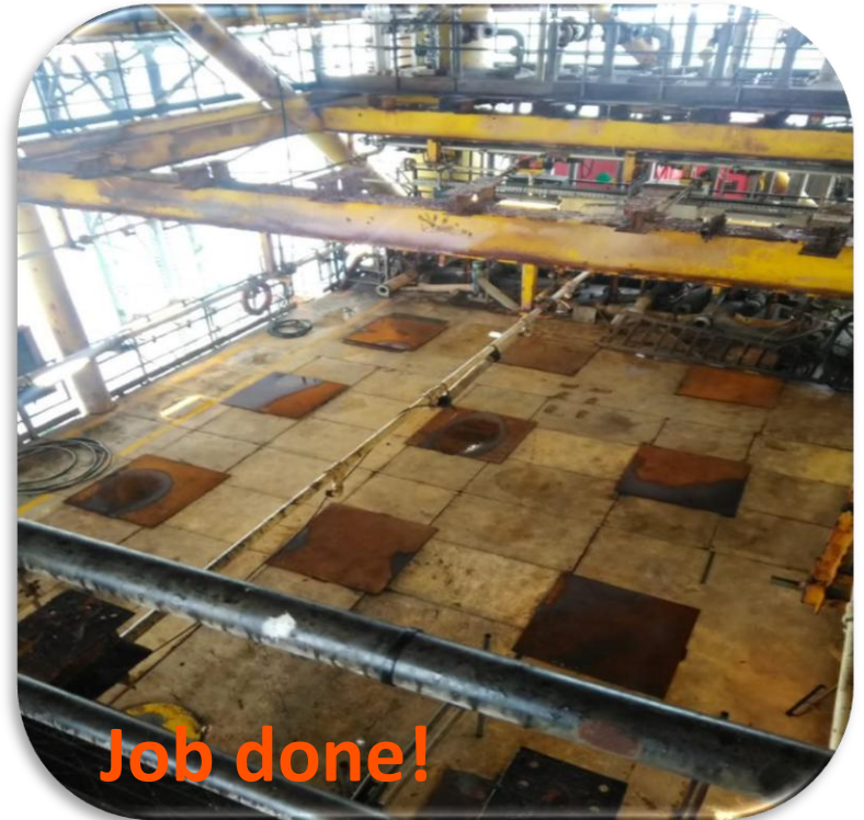
Schooner Platform, SNS (well bay following successful P&A campaign)
