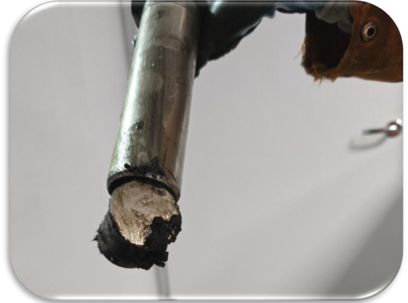
Gate valve milling to gain well access (recovered coupon)
