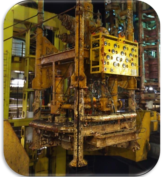
Recovered National SSXMT installed in 1979 c/w newly installed ROV panel
