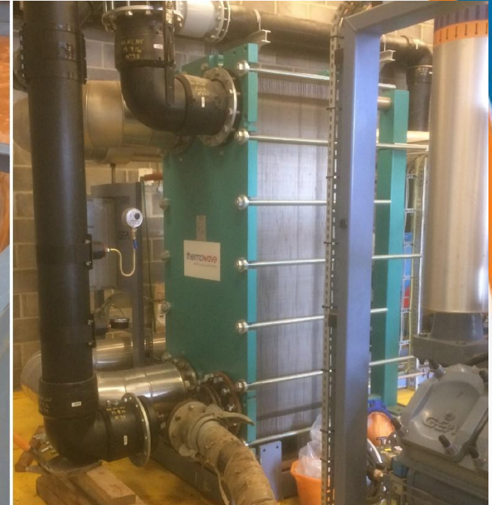
Circulating citric acid solution to remove ochre scaling from the plate heat exchanger at Abbotsford Road. Photo by © David Banks
