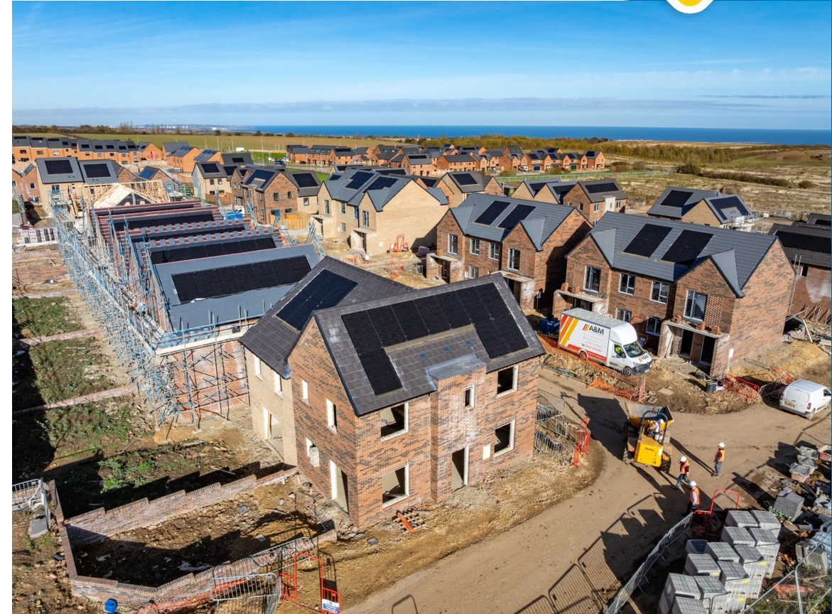
750 social homes under construction
