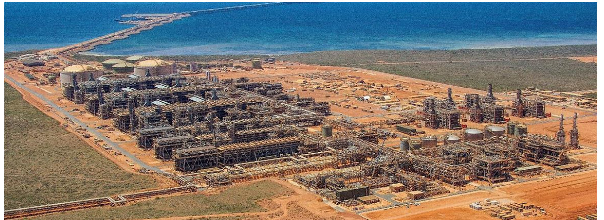
Gorgon LNG plant, with domgas and CO 2 compression /injection facilities
