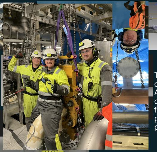
Tie-in of a new gas reservoir discovery in the North Sea. The AOGV is used to avoid shutdown of the producing wells. AOGV will facilitate 22 tie-ins of a new production reservoir to the existing process facility.
