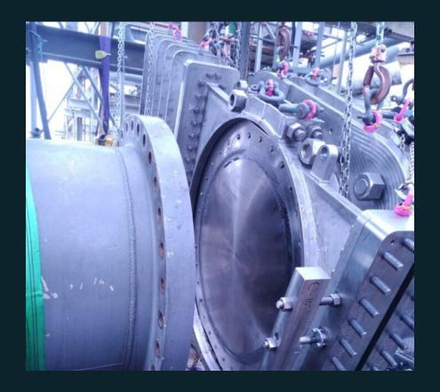
A 36" butterfly valve on the flare line of a major onshore LNG plant had been stuck in closed position for several years, preventing use of the backup flare system. The valve needed replacement without disturbance to the plant operation. A partial facility shutdown was planned as part of the normal facility maintenance routines and use of the backup flare system was critical to avoid a full shutdown. The AOGV prevented a full shutdown with one month's loss of production.
