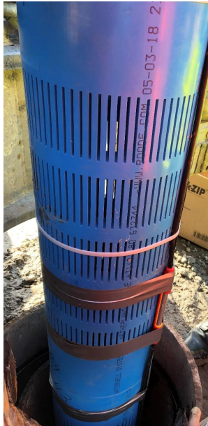
Screened interval being installed with electrical resistivity sensor
