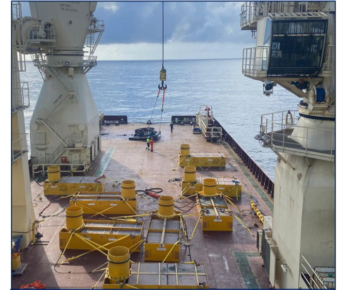
Temporary Guidebase and gravity base assemblies recovered
