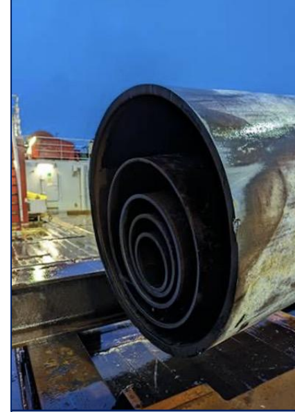
World first – 5 casing strings/single cut (Claxton)
