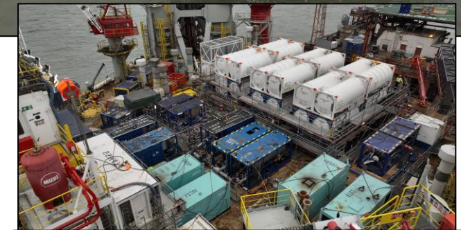
CO 2 loaded on rig, from Perenco CCS communication
