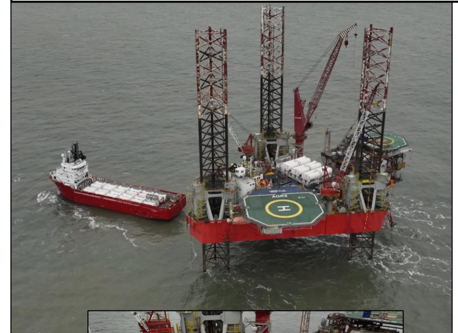
ERDA rig attached to Leman 27H platform, from Perenco CCS communication
