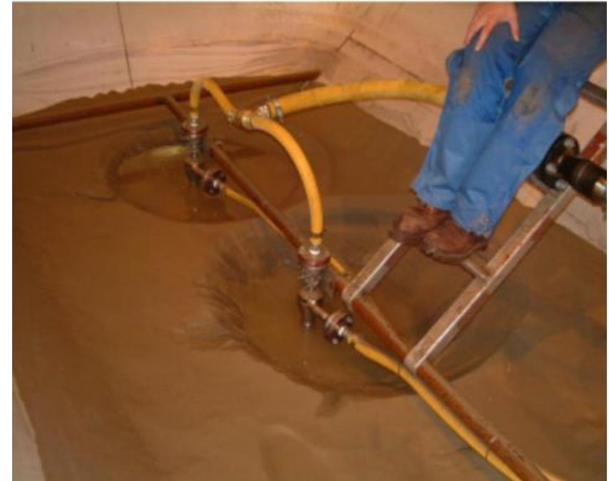
Sand in separator on Gullfaks C prior to implementation of next generation cyclone technology from FourPhase
