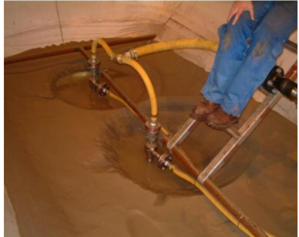
Separator filled with sand – Gullfaks C
