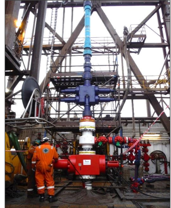
Slick line Rig Up
