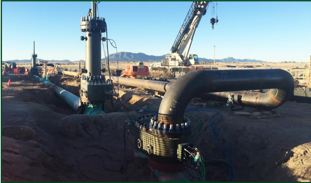
Kinder Morgan – 30" 148barg Liquid CO2 Bypass Maintaining Production
