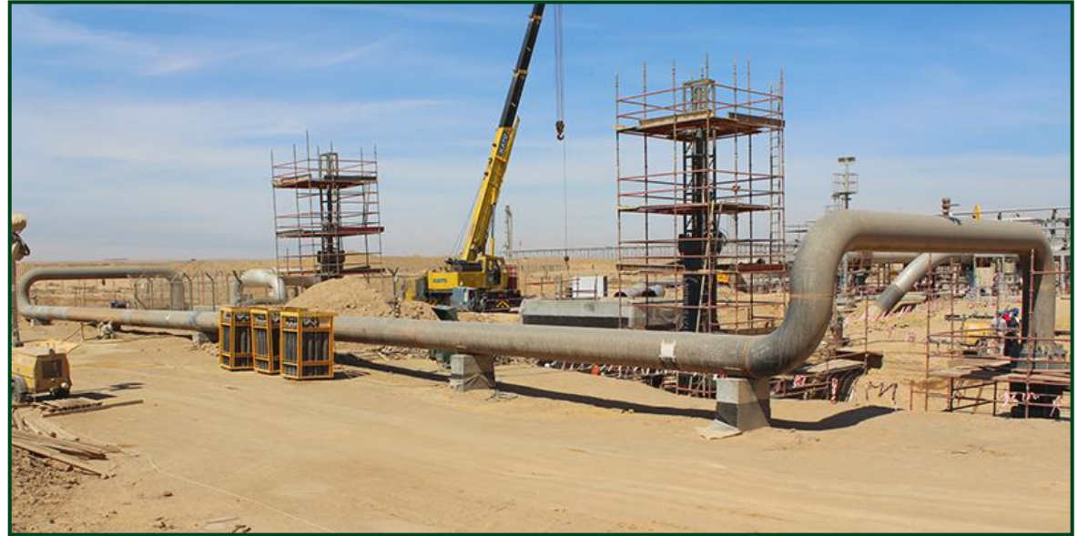
Kuwait Oil Company – 42" 30barg Gas Pipeline
