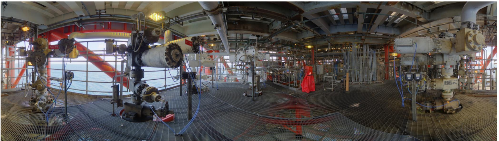
Erskine Normally Unattended Installation - Well Bay
