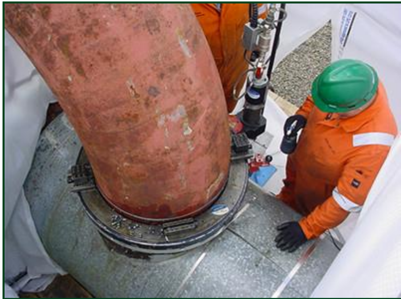
Pipe Cutting & Weld Preparation
