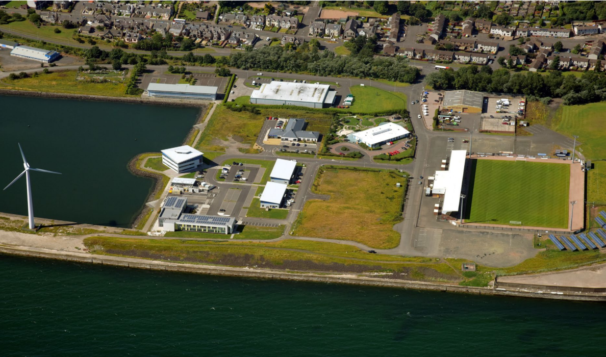
Levenmouth Community Energy Project
