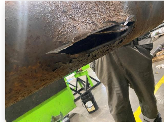
Test cut done prior to load out
