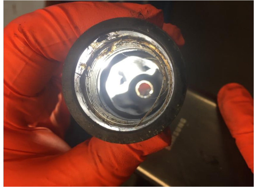
No evidence in scale inside the barrier check valve.
