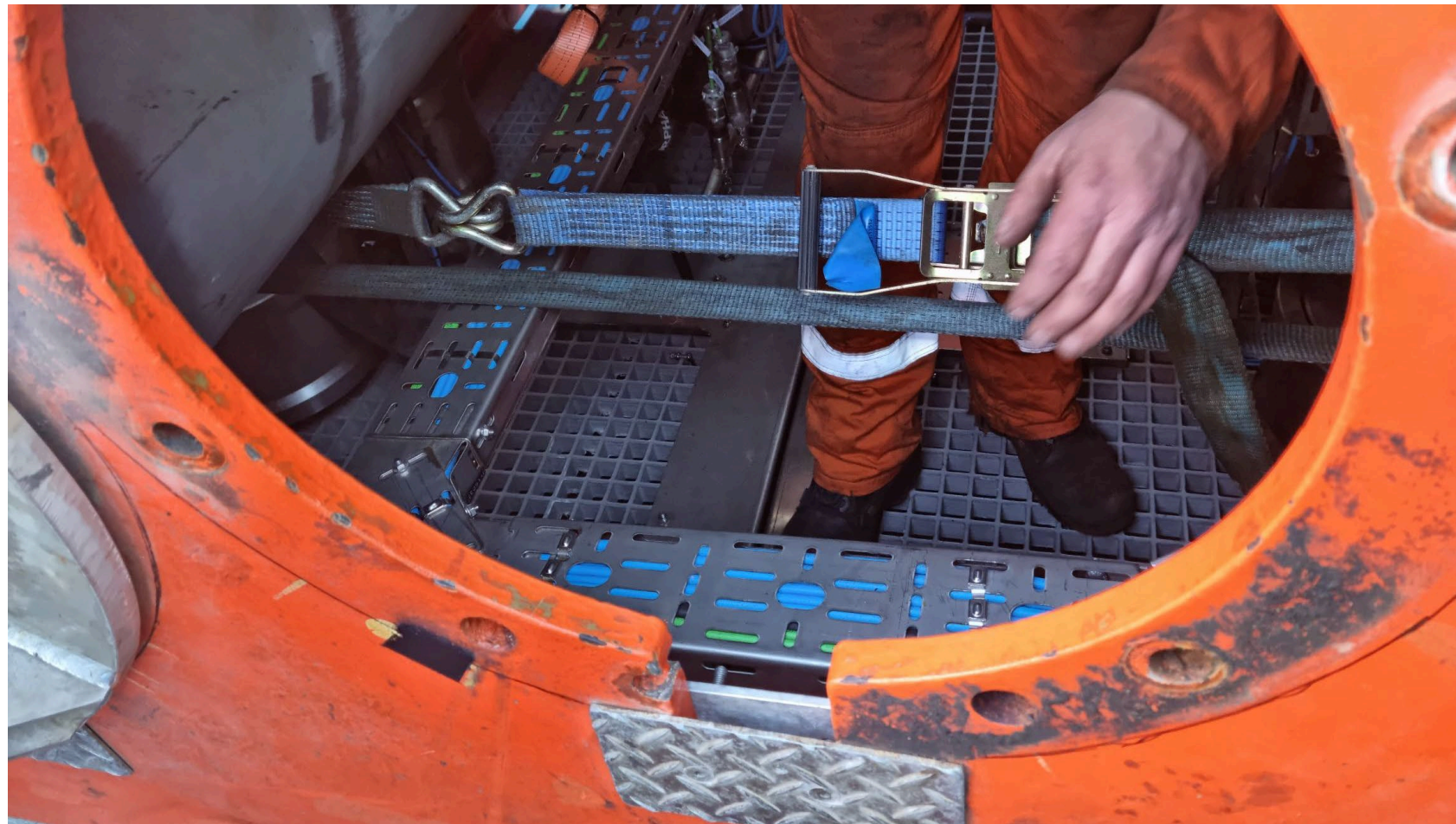
Removed one cyclone vessel of the DualFlow unit so under 8tonne crane capacity
