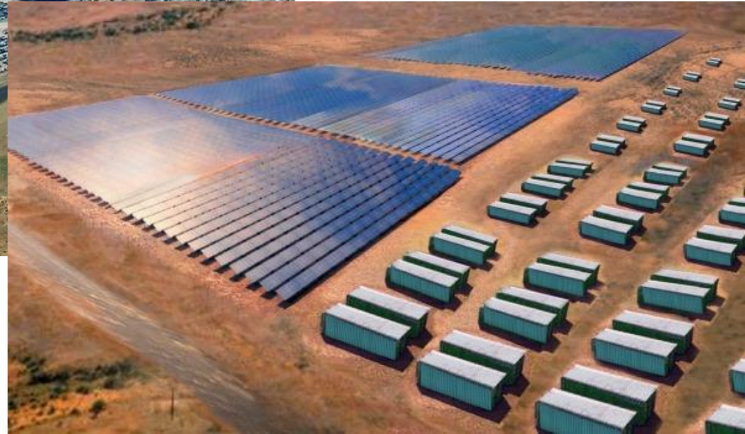
Riverland Solar Storage – South Australia 330 MW solar farm linked to a 100 MW/400 MWh battery installation
